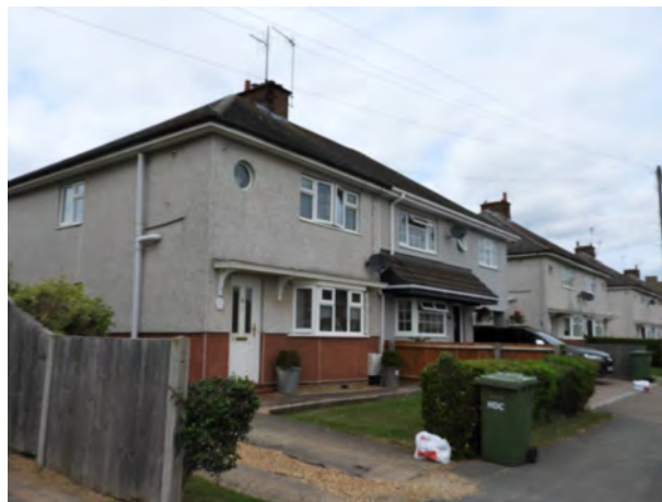
Station Road interwar semi-detached properties
