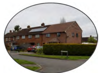
New build on Mandeville Road
