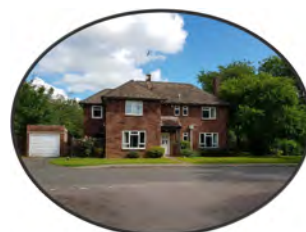
Married Quarter along South Road
