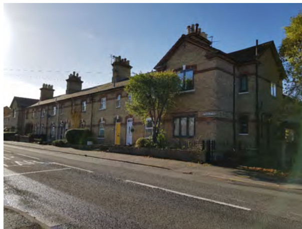
Terraces located along Stukeley Road
