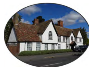
The Old Manor House, 66 Hartford Road
